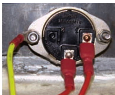
Fig B: Thermostat Connection
